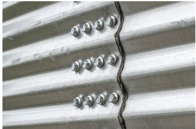
Grade 8.2 bin bolts are used throughout to ensure strengths and stability. Roofs and lighter gauge sidewalls use 5/16" (0.79 cm) bolts. Heavier gauge sidewalls use 3/8" (0.95 cm) bolts.
