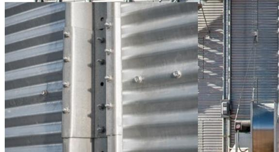
**12 gauge splice** ensures that stiffeners are properly butted to effectively transfer sidewall load to the foundation.
