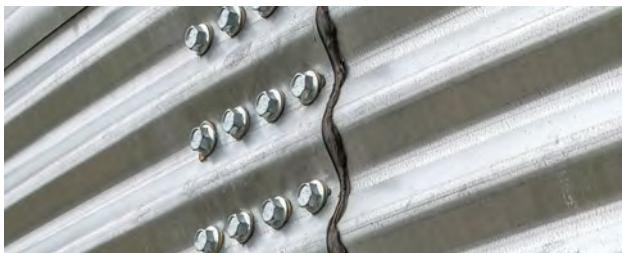
**Grade 8.2 bin bolts** are used throughout to ensure strength and stability. Roofs use 5/16" (0.79 cm) bolts and sidewalls use 3/8" (0.95 cm) bolts.
