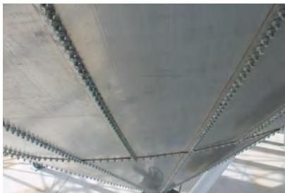
**Galvanized panels** ranging from 12 gauge to 8 gauge Grade 50 are designed to withstand hoop and top tension loads throughout the range of sizes available. Cross braces keep tank evenly braced during loading.
