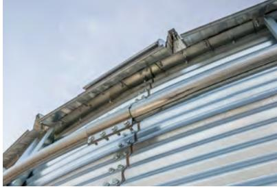
**Heavy duty wind rings** are easily attached to the stiffeners on bins requiring this extra measure. Pre-punched wind ring holes and special attachments simplify installation.
