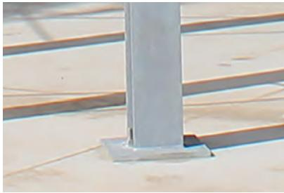
**Heavy base plates** welded to the bottom end of the support columns provide a positive attachment to the concrete foundation with proper anchoring.
