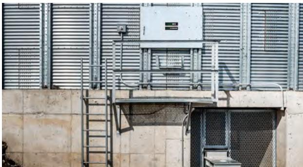
**One ring door** in sidewall provides full and easy access regardless of door option selected.
